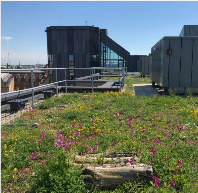
Biodiverse extensive green roof, David Attenborough Building, Cambridge, England (© Green Infrastructure Consultancy)
