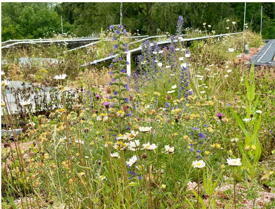
Figure 1. Noah´s Ark, combining wildflowers and solar panels to a biosolar roof.
