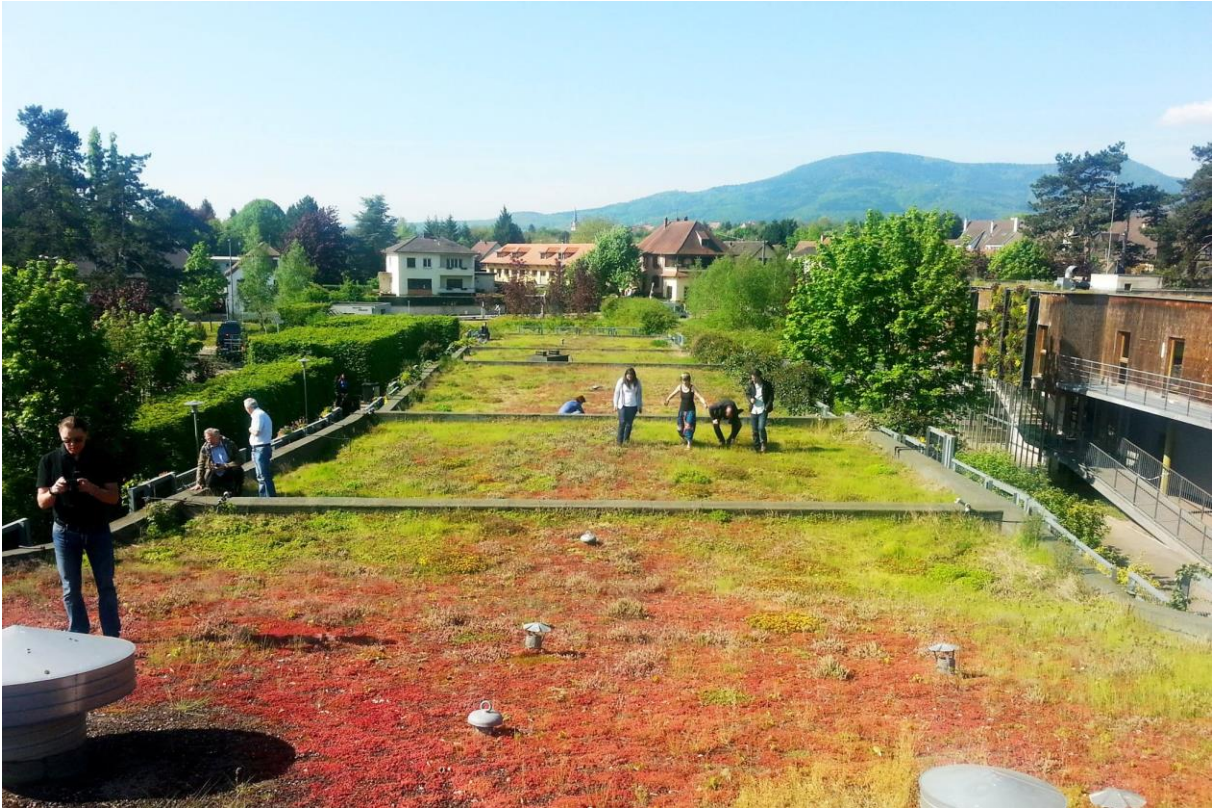
Figure 11. Green roof and wall experts excursion on a school building in France.
