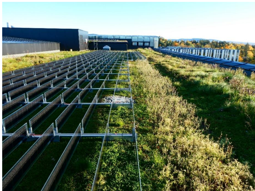
Figure 3. Vertical bifacial panels on an Oslo office building.
