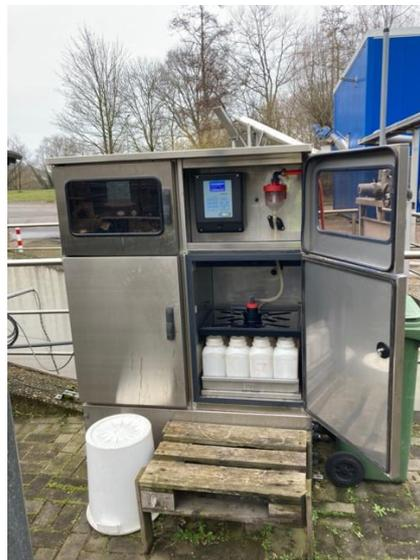
*Figure 9 -Automated Sampling Device at the WWTP Aachen Soers (courtesy of F. Joerens, Wasserverband Eifel-Rur)*
